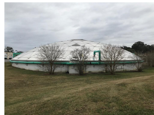
TRICKLING FILTER NO. 3
