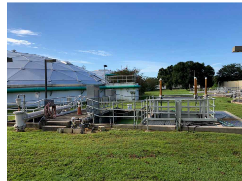
TRICKLING FILTER EFFLUENT SPLITTER BOX
